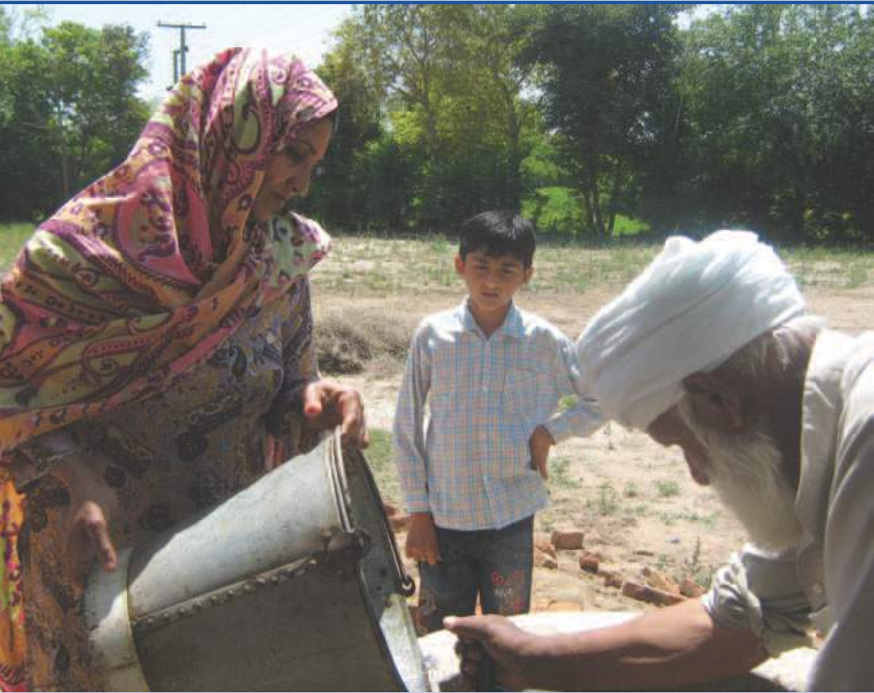
Husband and wife in Pakistan have both received the biogas user training and are feeding the biogas plant together
